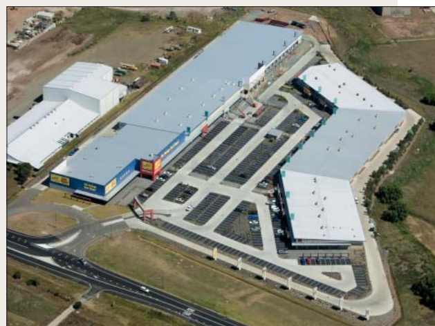
Hunter Supa Centre – nearing completion.
